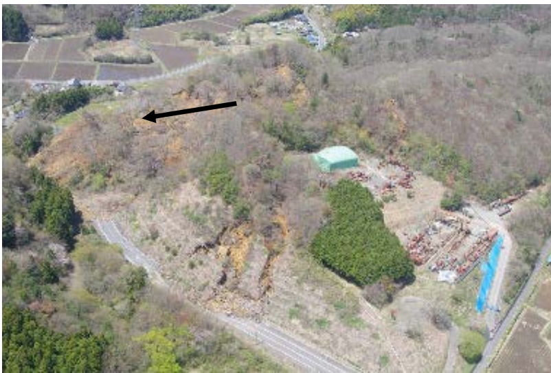
Fig.4 A deep-seated slide blocked a highway in Iwaki
