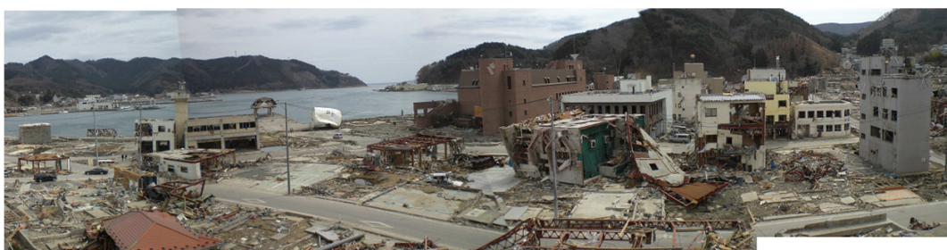
Fig.3 Devastated port town of Onagawa (April,3 2011) Three-storied buildings even fell down.
